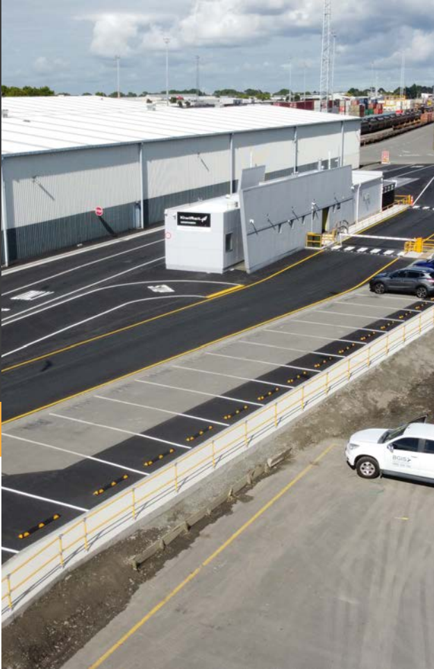
03 KIWI RAIL – CONTAINER TERMINAL PAVEMENT UPGRADE
