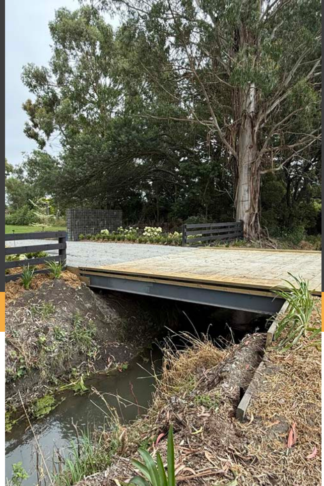
04 TAI TAPU ROAD SAFETY AND PAVEMENT WORKS
